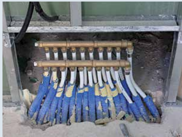
Fig. 9-13 Colectores
