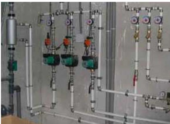
Figure 9-2 tube multicouches
